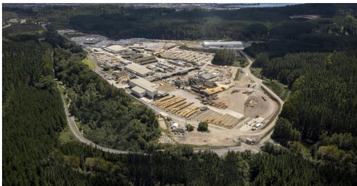
Pictured: Red Stag Timber sawmill in Rotorua processes 8,000 individual logs per day.
