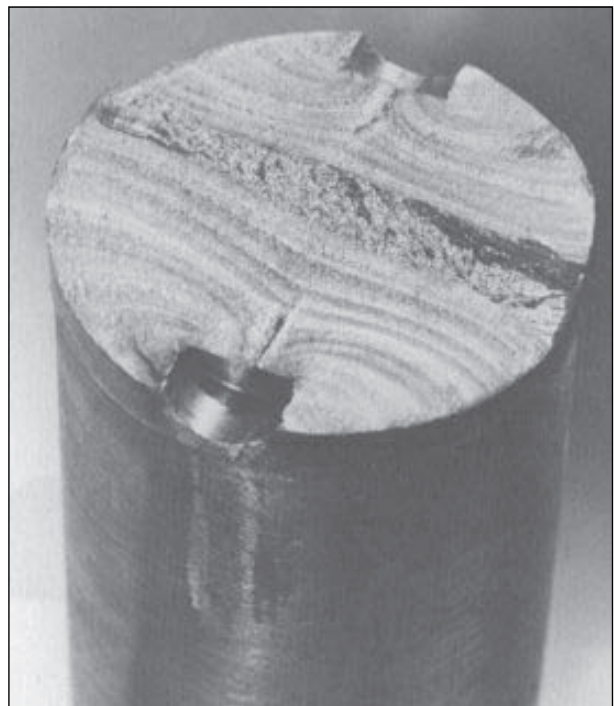
Failure started at the keyways where the transverse cracks grew to be so large that the remaining material could no longer sustain the load and the shaft finally broke. Note the shiny surface from the keyways to the break, which is granular in appearance.
